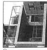
Clear Louvers with solid frame Clear Glass with solid frame, color equal to Dulux Outdoor Cladding - Clear Powder Coat Finish
