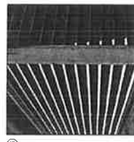
Fixed Aluminium Louvers - Horizontal Clear Glass with solid frame, color equal to Dulux Outdoor Cladding - Clear Powder Coat Finish
